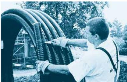
1. Place the CALPEX-ring at the start of the line, and cut the outermost fixing tape.
