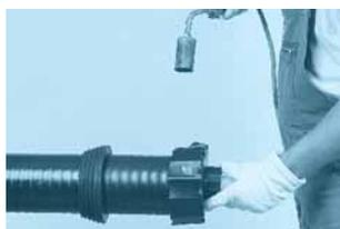
8. Carefully put end cap CPX for below ground onto the pipe according to the enclosed Raychem DHEC installation instruction or attach end cap CPX for above ground.
