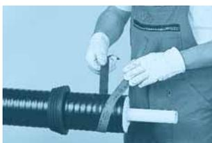
7. Grind protective sheath.
