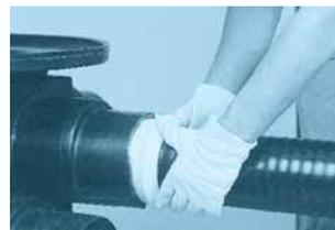
3. Fit the two-section reducer ring (only needed for CPX dimensions 76, 91 and 126 mm).
