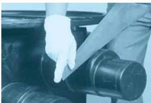
1. Saw the shaft mouth to match the outer diameter of the pipe – Ø 136, 166 or 186 mm are possible.
