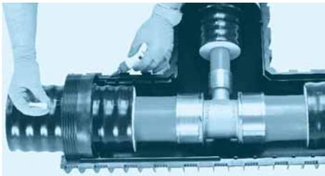
5. Clean all gluing surfaces so that they are free from grease, then apply a continuous line of adhesive, about 4 mm (1/8 inch) wide, to the lower shell only.
