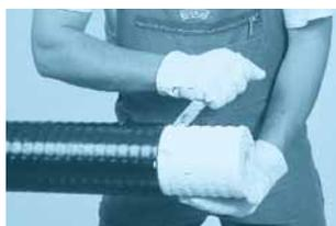
5. Cut back insulation over the marked distance.
