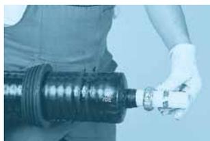
1. Put the union nut and the clamping ring onto the pipe.
