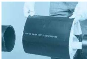
2. Pull the shrink hose over the pipe ends.
