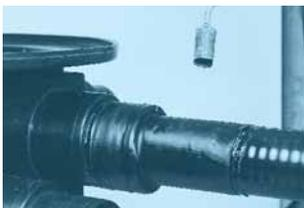
5. Remove the protective film from the shrink hose and heat-shrink.
