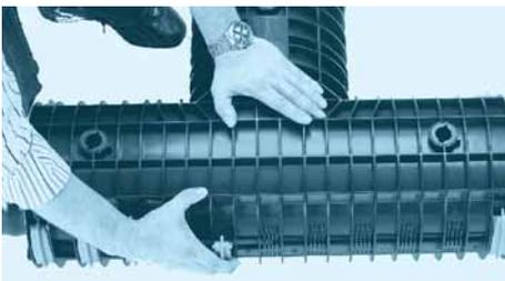
7. Immediately apply all the clamps at the positions provided for them, and allow the glue to harden for **20 minutes**.
