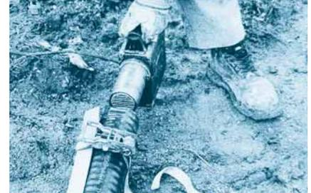
3. Use hot air or hot water to heat the medium pipe; let it cool – and the job is finished.
