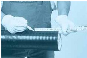
1. Mark the distance (x, y, z) + 1 cm from the end of the pipe.
