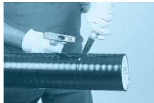
3. Open the jacket longitudinally. Knife max. 5 mm deep into foam.
