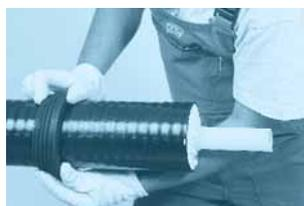
6. Mount the wall seal. Stretch the clip (if existing).
