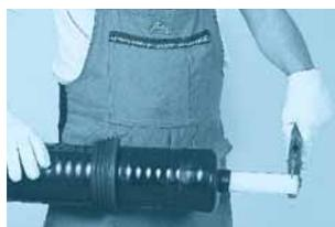
9. Cut the PEX-Pipe square to its axis (max. 1 cm).
