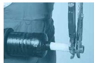
4. Move the union nut, the clamping ring and the muff together, and tighten them adequately. Caution: Do not overtighten!
