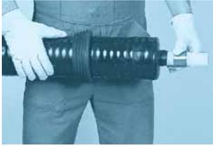
1. Push the sliding sleeve over the pipe; the inner ridge must point to the end of the pipe (with the conical end of the sliding sleeve towards the end of the pipe).
