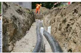
Delivery lengths up to 810 metres on one coil and highly flexible pipes simplify routing. Short construction times and small trenches minimise construction costs.
